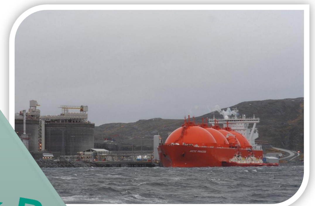
LNG-Terminal Melkøya, Tanker Arctic Princess Quelle: www.statoil.com
